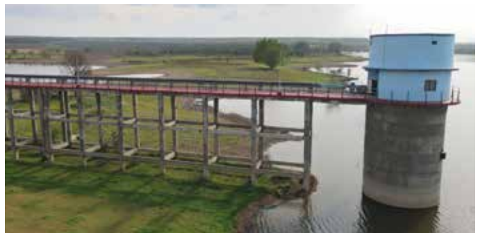
Approach Bridge constructed for a length of 588 meters and width of 4.20 meters at Intake well in Gadakota Multi Village Rural Water Supply Scheme in Sagar District in Madhya Pradesh.
