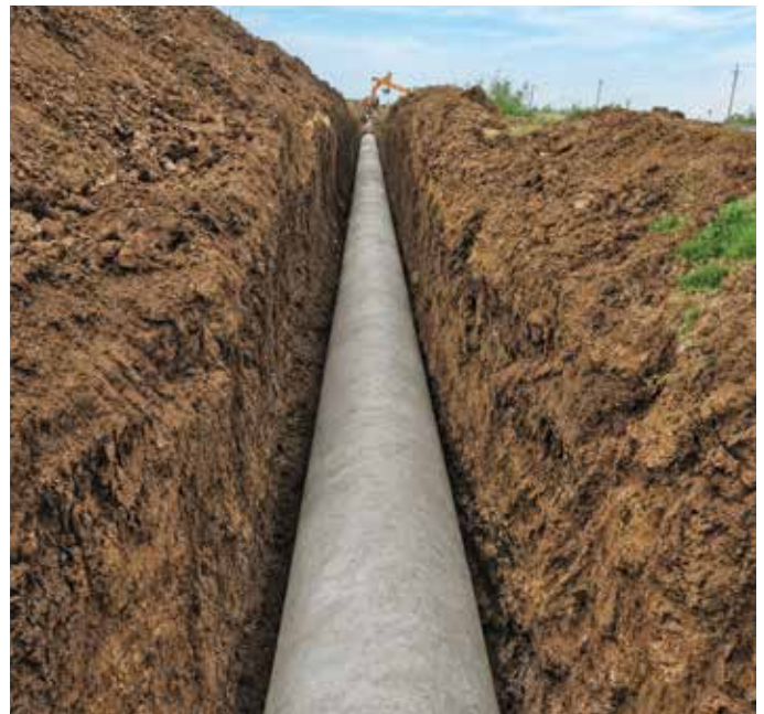
1250 mm dia MS pipeline laying at Kushtagi MI & GWDD project in Karnataka
