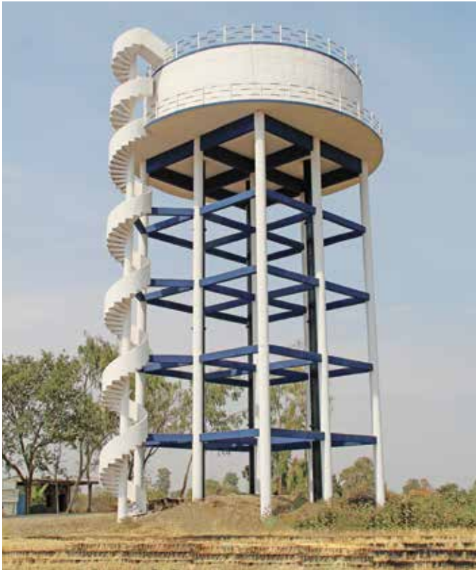
3.6 lakhs Ltr. capacity Break Pressure Tank (BPT) at Buldhana Water Supply Scheme, in Maharashtra
