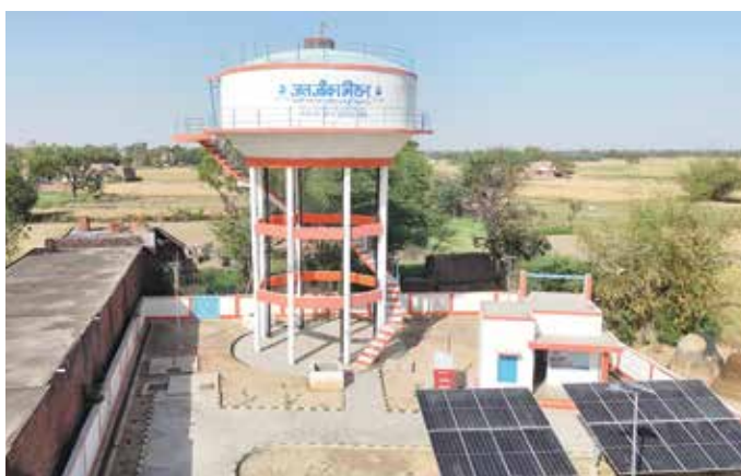
Tube Well cum Pump House, 20 KW Solar Power Plant and 300 KL Over Head Tank at Etaili Village, Auraiya District for Kanpur Water Supply Scheme (SWSM) in Uttar Pradesh.
