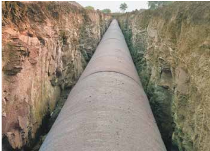
1800 mm dia PCCP pipe line laying work at Sulwade Jamphal Kanoli Lift Irrigation Project, Dhule in Maharashtra.
