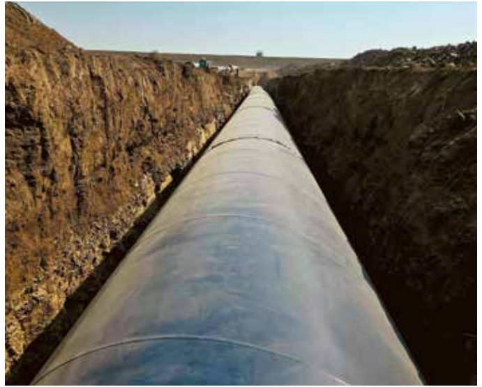
3200 mm dia M. S. pipe line laying work at Sulwade Jamphal Kanoli Lift Irrigation Project, Dhule in Maharashtra.
