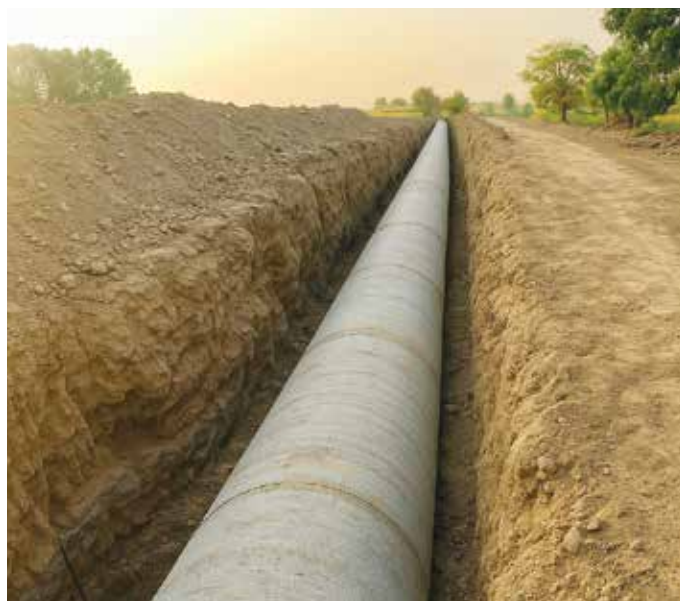
2000 mm dia PCCP pipe line laying for Varkhede Londhe Irrigation Project in Maharashtra.
