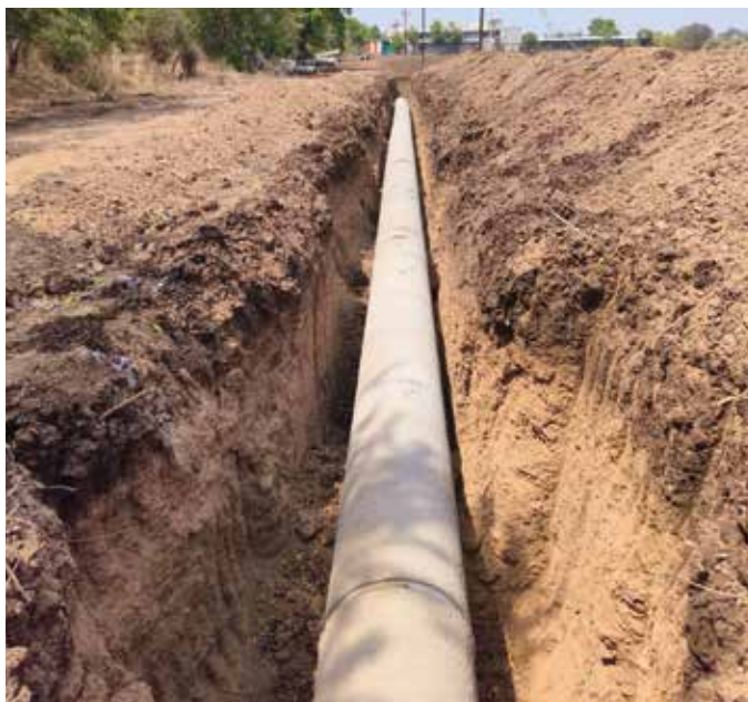
600 mm dia PCCP pipe line laying for Jalgaon Jamod and 150 villages Regional Rural Water Supply Scheme for Maharashtra Jeevan Pradhikaran in Maharashtra.
