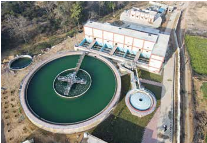
25 MLD Water Treatment Plant for Kuraicha Water Supply Scheme in Uttar Pradesh.
