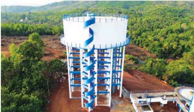
11.70 Lakh Liter Master Balancing Reservoir at Degave village for Tillari Water Supply Project for Maharashtra Jeevan Pradhikaran, in Maharashtra.
