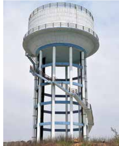
850 KL Overhead Service Reservoirs at Kandaila Multi Village Rural Water Supply Scheme in Rewa District in Madhya Pradesh.
