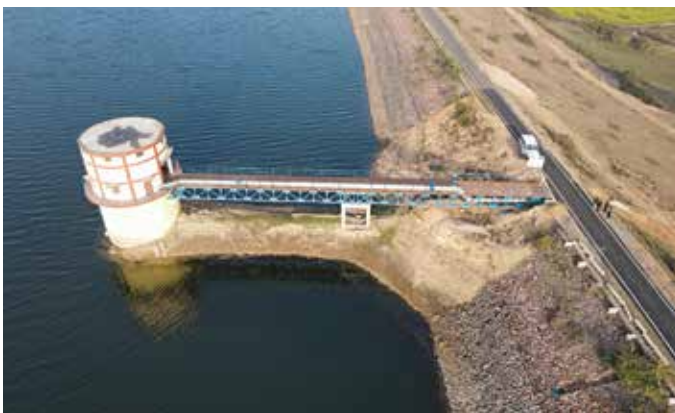
Intake Well cum Pump House at Saprar Dam for Kuraicha Water Supply Scheme in Uttar Pradesh
