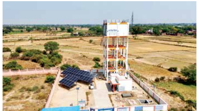
Tube Well cum Pump House, 20 KW Solar Power Plant and 150 KL Over Head Tank at Bhagautipur, Auraiya District for Kanpur Water Supply Scheme (SWSM) in Uttar Pradesh
