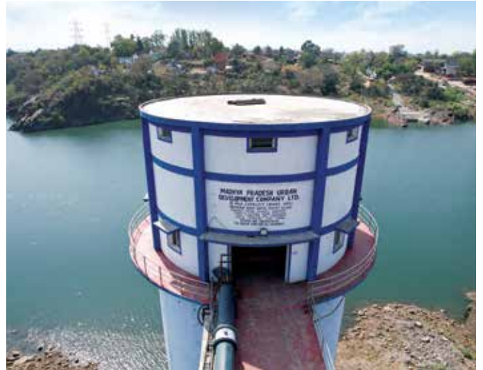
27.93 MLD Intake well cum pump house at Bhedaghat Town for Bhedaghat Water Supply Scheme in Madhya Pradesh.
