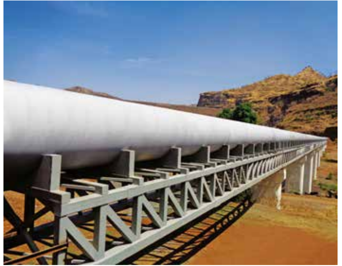
1500 mm dia MS pipeline laying at Chilhowadi Pipeline Project, in Maharashtra
