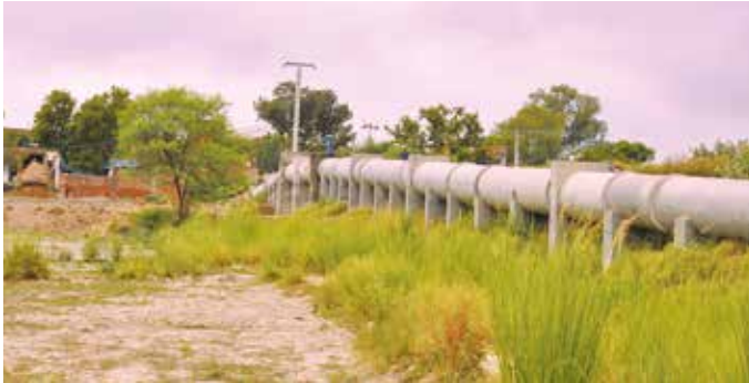
1200 mm dia BWSC pipeline at Santhi Village for Firozabad WSS, in Uttar Pradesh.
