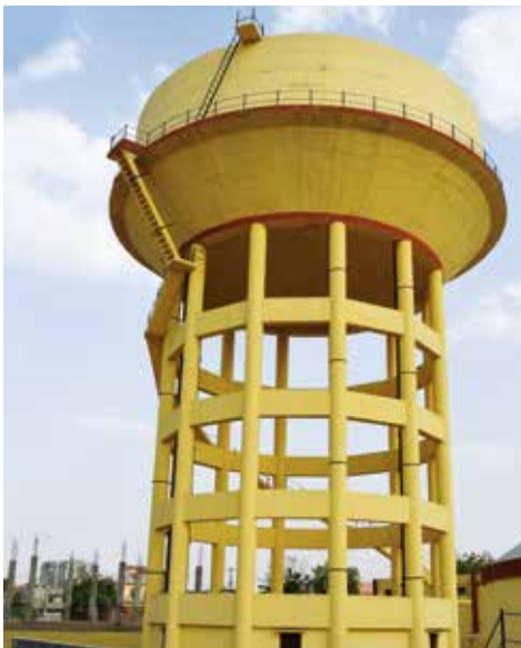
2000 KL OHSR for Urban Water Supply Scheme, Alwar, in Rajasthan
