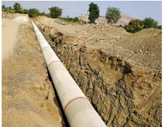
1300 mm dia PCCP pipeline laying at Chilhowadi Pipeline Project, in Maharashtra
