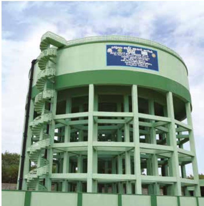
17.50 Lakh Litre Capacity Balancing Reservoir at Sundamedu for Tiruppur Water Supply Scheme, in Tamilnadu.
