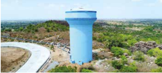
400 KL OHBR at Balkonda Hillock for Balkonda (TDWSP) Project, in Telangana.
