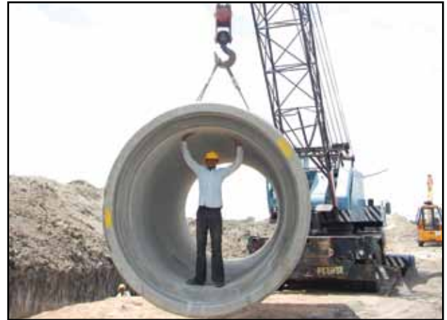
2000 mm dia PSC pipe for Pulikanuma Lift Irrigation Scheme (A.P)
