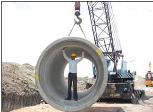
2000 mm dia PSC pipe for Pulikanuma Lift Irrigation Scheme (A.P)
