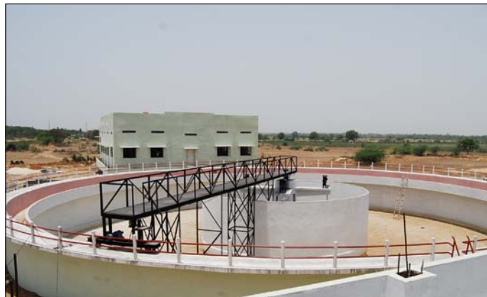
Clarifloculator at Gajwel Phase-I Project.
