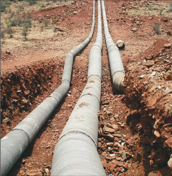
1000 mm & 600 mm dia M.S. Pipe lines for J. C. Nagi Reddy Drinking Water Supply Scheme, Phase II & III, Ananthapur District, Andhra Pradesh.
